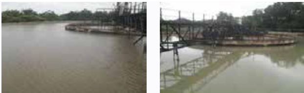
Sewerage Treatment Plant (STP) at Degaon
